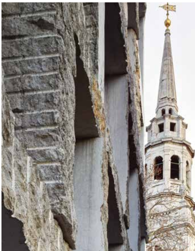
Far left The main east elevation of 15 Clerkenwell Close shows the curious limestone exoskeleton with its various surface treatments.
