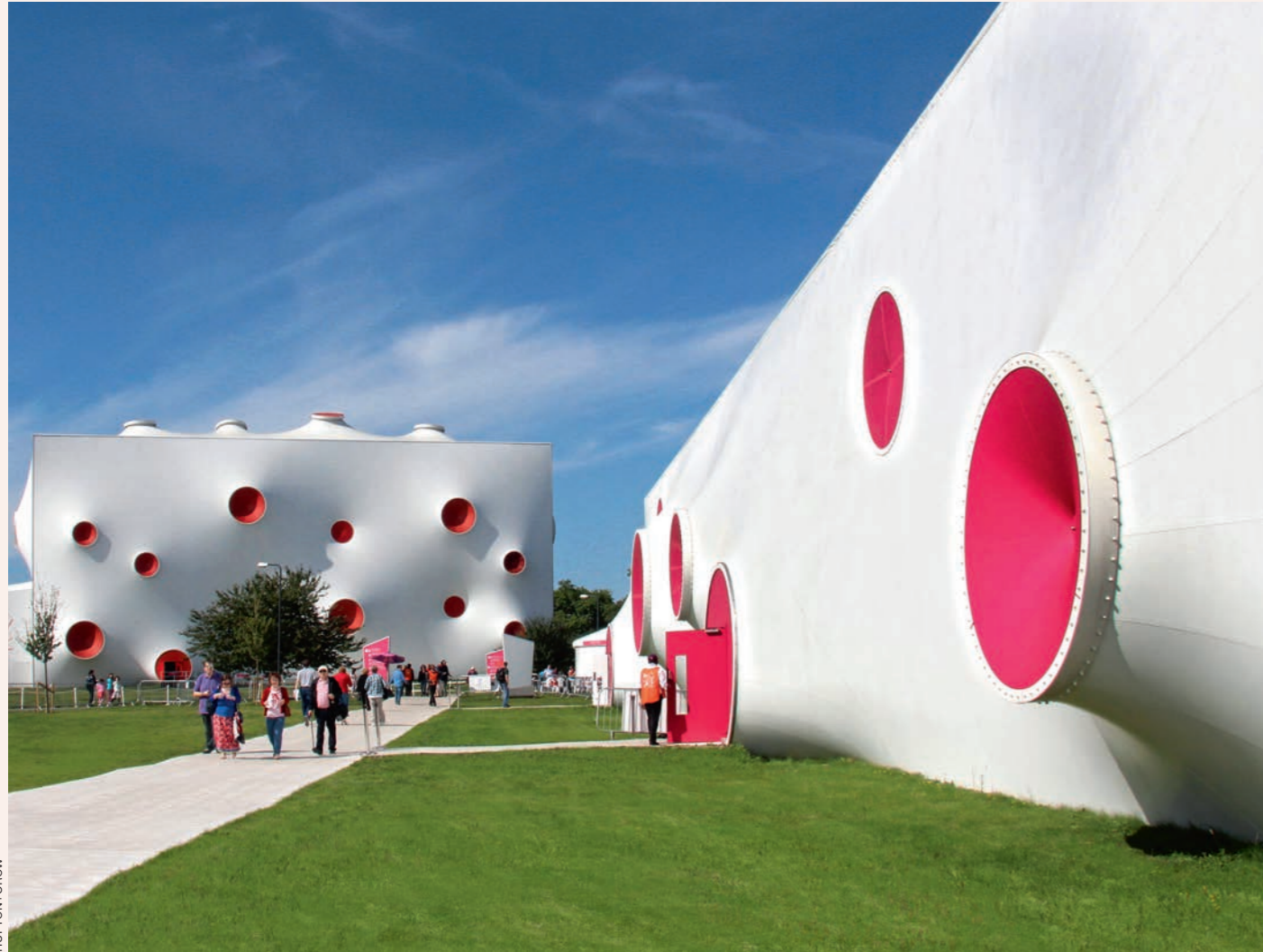
Below Magma Architecture's bold, temporary, PVC-covered shooting venue for the London 2012 Olympics.
